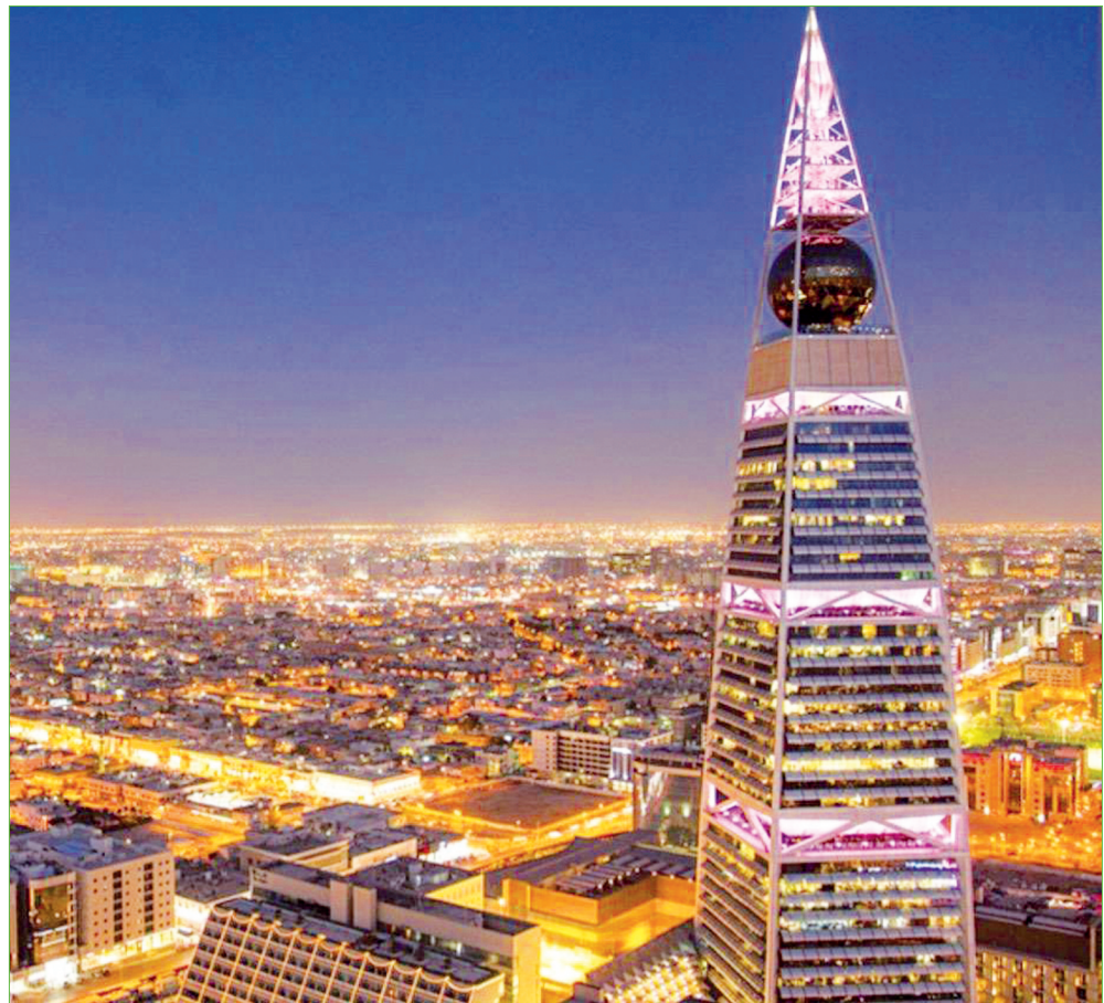
Al Faisaliah Tower, Riyadh
